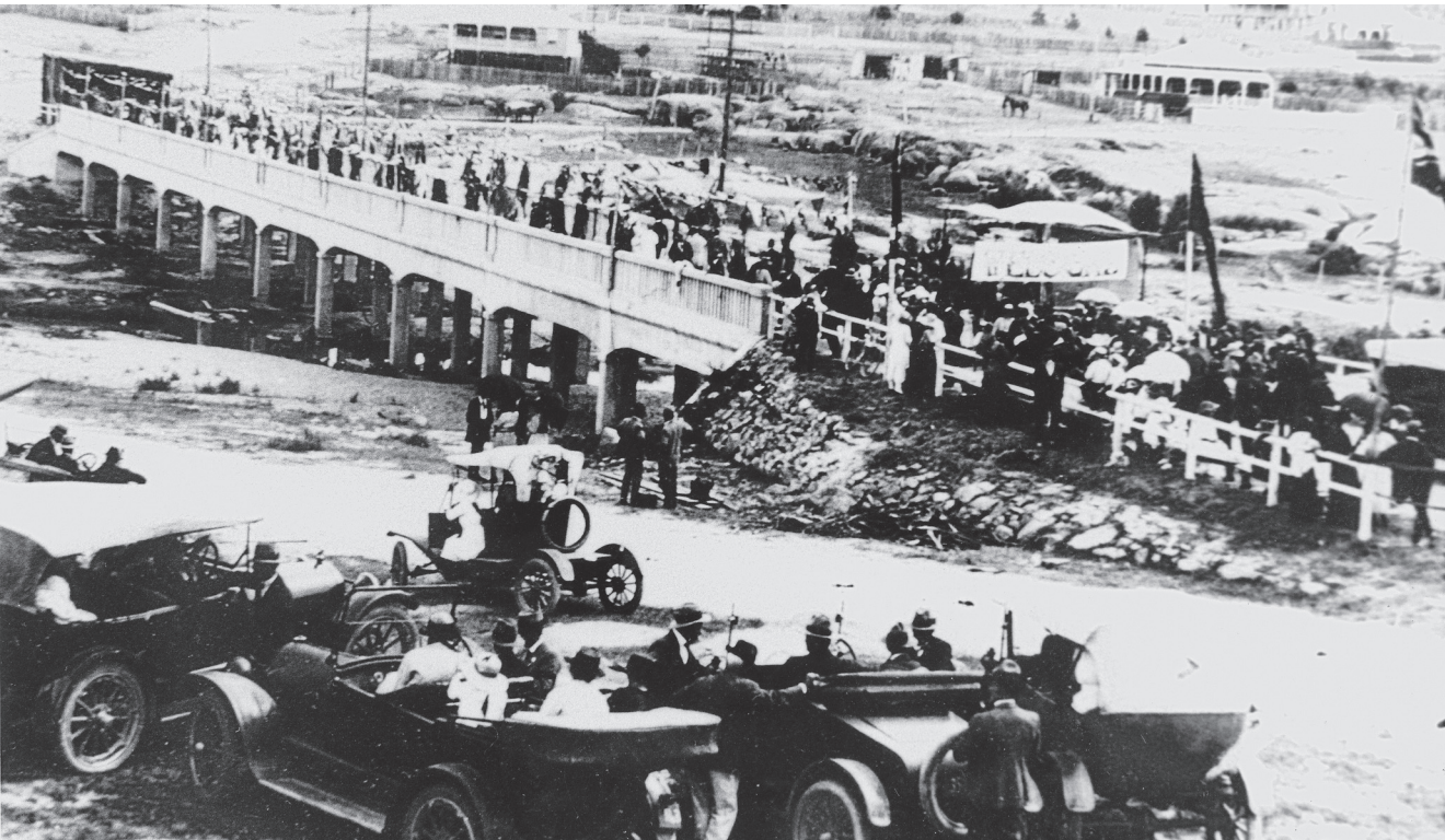
Carnarvon Bridge. (SDRC from State Library of Qld)
